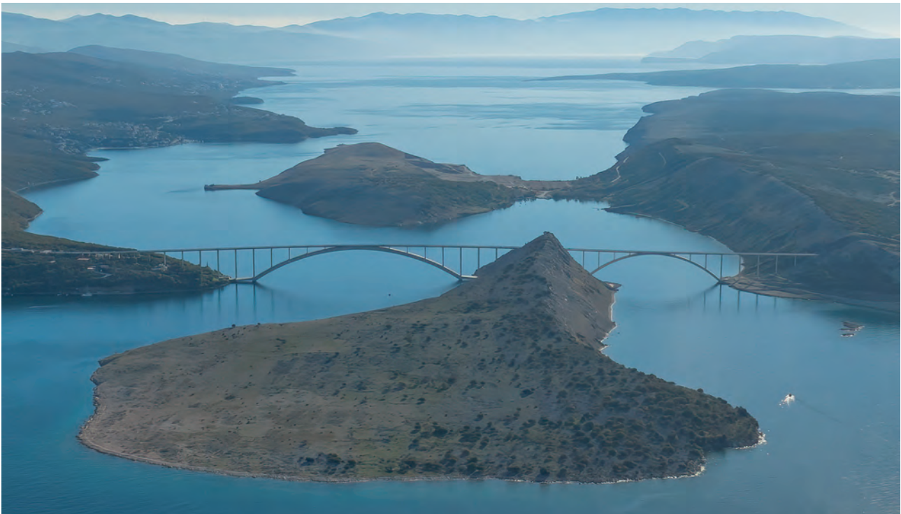
Tihi Kanal, channel (from NW)
